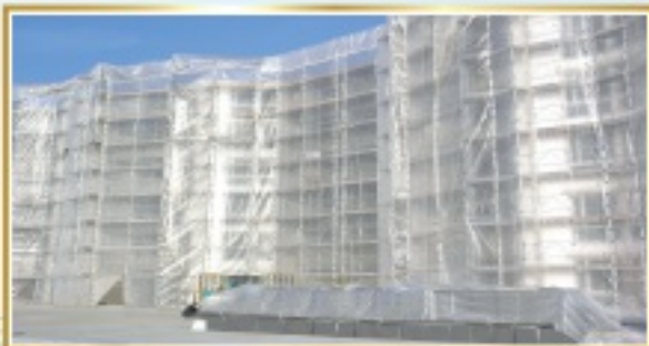
Building Construction Coverage
