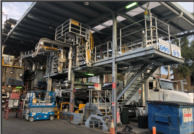
Bitumen loading application in Sydney, Australia
